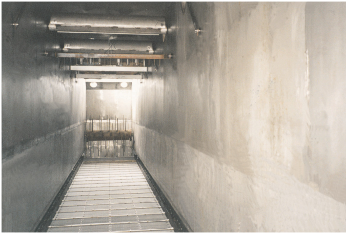
Inside view towards discharge end
